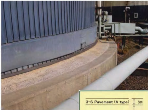
Sulphur tank foundation in Tomakomai city, Hokkaido Idemitsu Kousan Co., Ltd Temperature: 150°C Construction date: Jul, 1984 Area: 280cm 2
